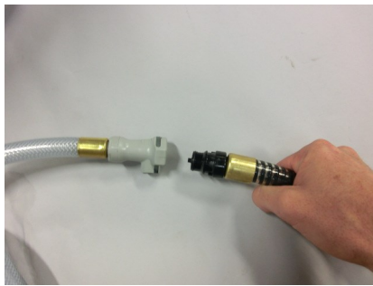
Attaching intake service hose to hose to sea strainer.
