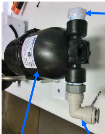
PL-SWF-1/2x1/2 1/2"NPT x 1/2" Tube John Guest swivel elbow
